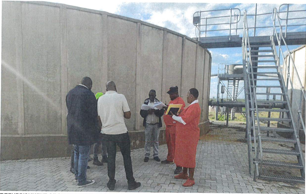
REFURBISHMENT OF SEWER TREATMENT PLANT IN SWARTDAM
